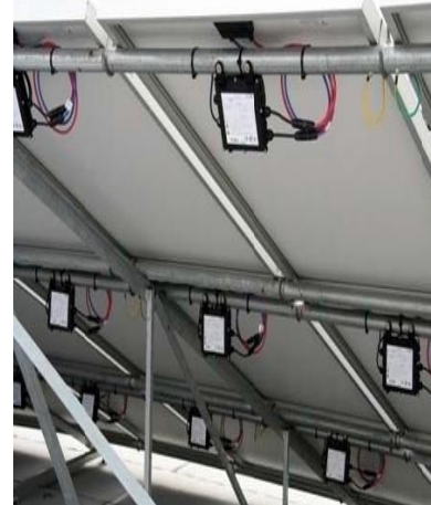
Typical system wiring
